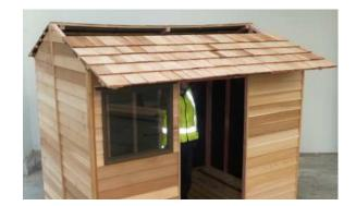
Step 15:Using 75mm tek screws, screw roof panels into end wall panels, (2 screws per panel), ensuring end of rafter lines up with centre of gable panel.
