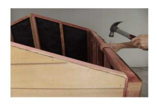
Step 10: Using 30mm clouts nail top cedar boards to stiffeners (2-3 per board). Predrill holes to stop boards from splitting.
