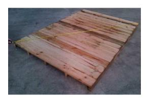
Step 3: Nail plastic weather strip to edge of floor on all four sides, with 30mm clouts, (approx 5 nails per side) ensuring top edge is flush with top of floor. This isn't required if shed is on a concrete base.
