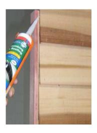
Step 7: Silicone and nail remaining beads on each panel. Screw panels together using 3 tek Screws per join and 4 on the longer joins on gable end panels.
